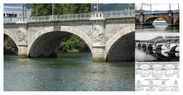
Designed by French engineers and completed in 1864, this example of the best stone bridge engineering has been restored according to FHECOR's design. Its 160 years of service are proof of the durability and sustainability of masonry bridges.
